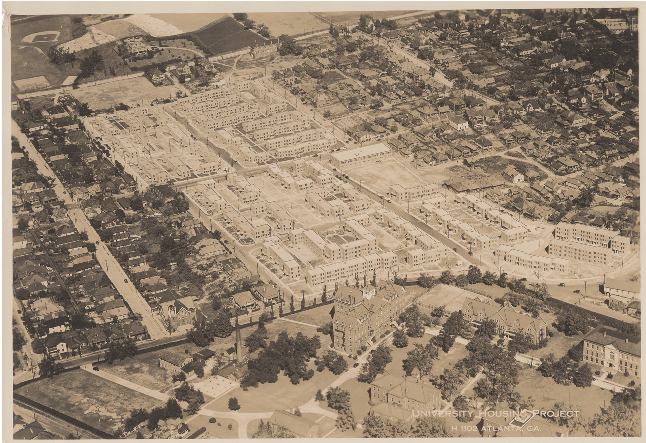
Figure 8 Edwards and Sayward (architects) with O. I. Freeman (engineer), University Homes, Atlanta, under construction, ca. 1936, aerial view showing blocks of wood-frame bungalows on the east and west, Spelman College on the south, and Atlanta University on the north (Charles F. Palmer Papers, box 167, folder 10, Stuart A. Rose Manuscript, Archives, and Rare Book Library, Emory University).
